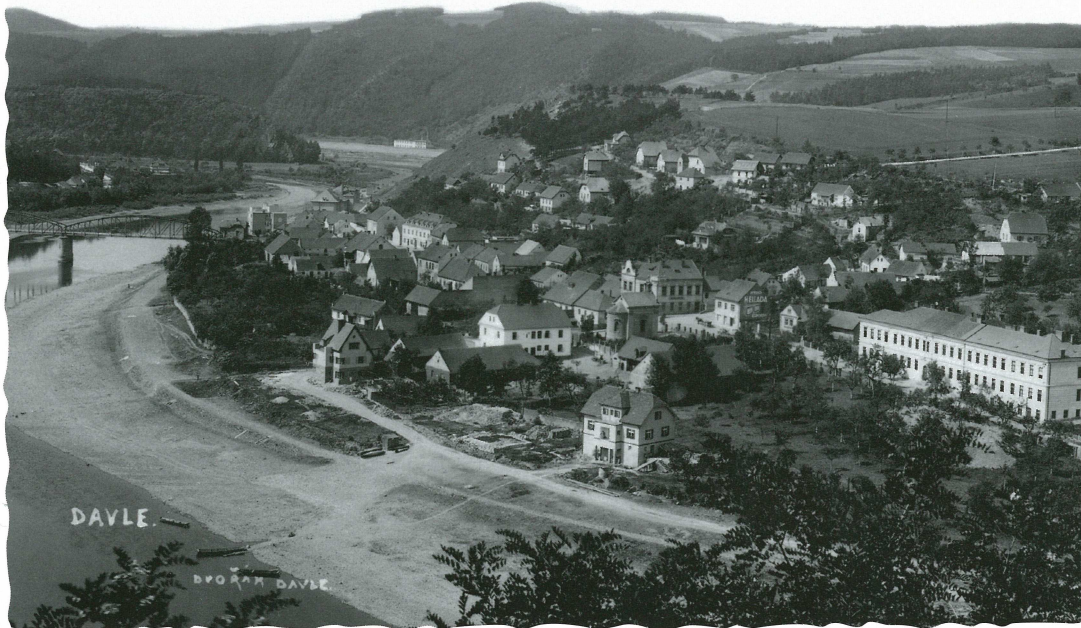
Davle in thirties; the iron bridge “played” in the film “The Bridge of Remagen” by Milos Forman 2
